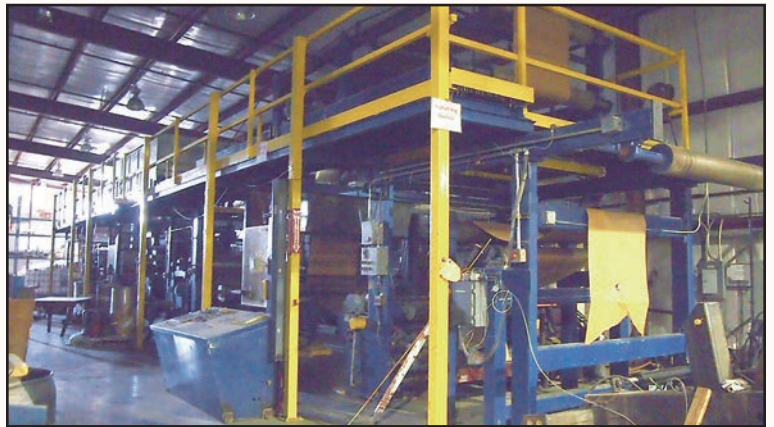
ASPHALT PROCESSING PLANT
